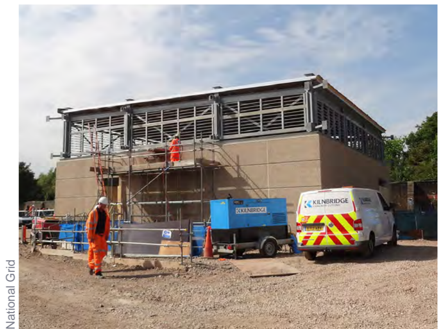
Example of a Tunnel Head House under construction
