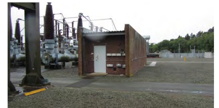
Existing relay room
